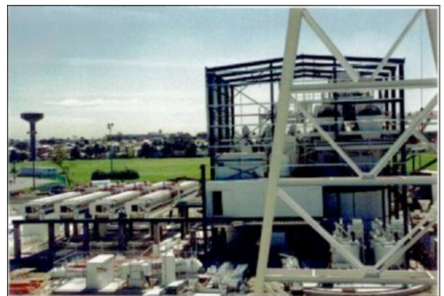
Sydney STP during erection
