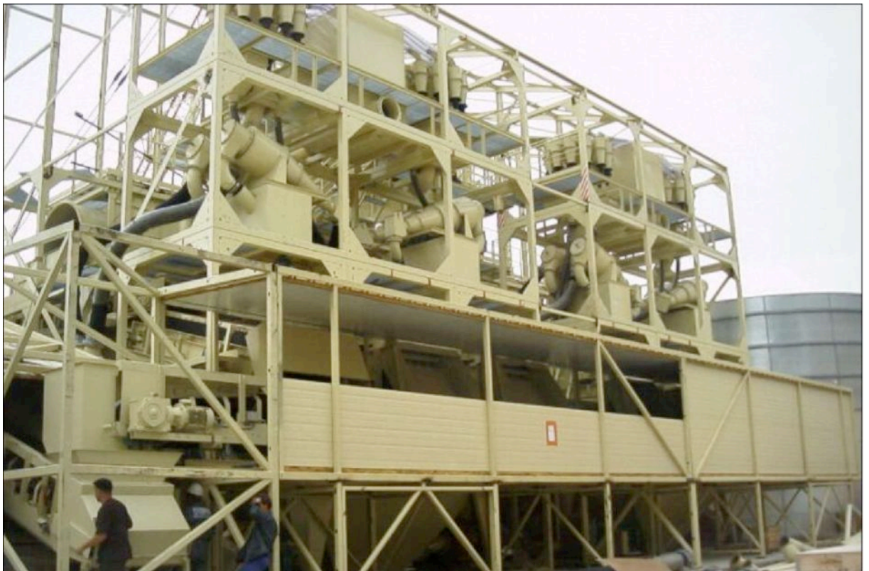
Lefortovo (Moscow) 2800 m 3 /h (during erection)
