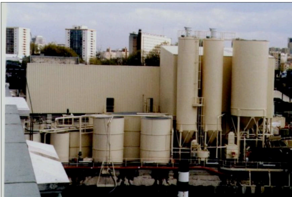
General view of IGCN plant with specific seepage water treatment
