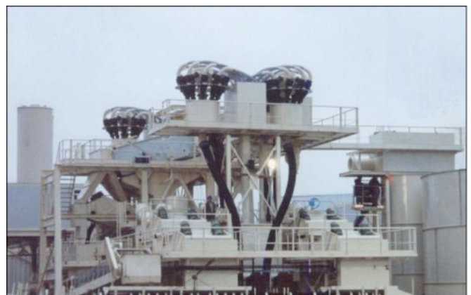
Sophia STP during erection
