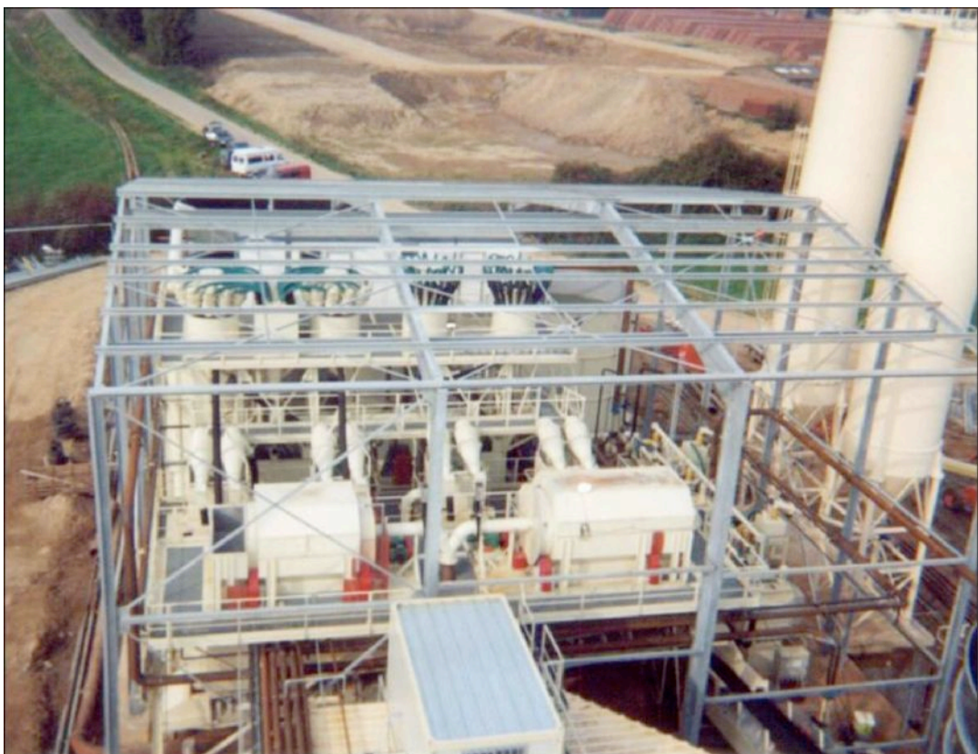
Pannerdensch Kanaal 1600 m 3 /h (during erection)
